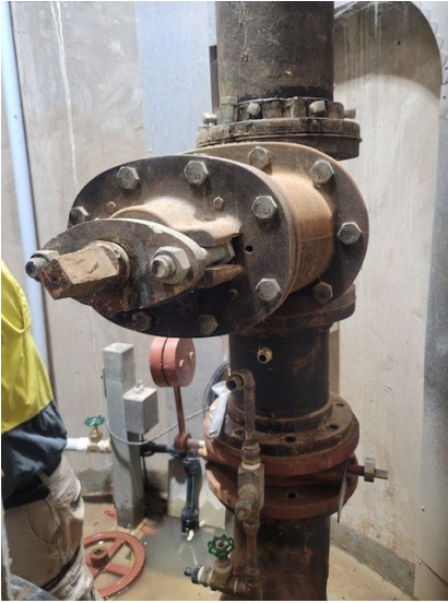
Change SV and non-return valves at No 2 Pump Murray St pumping station
