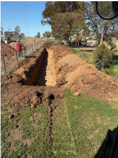
Booligal Rec Reserve Septic rubble drain being installed
