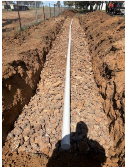
Booligal Rec Reserve Septic rubble drain being installed
