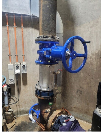
Change SV and non-return valves at No 2 Pump Murray St pumping station
