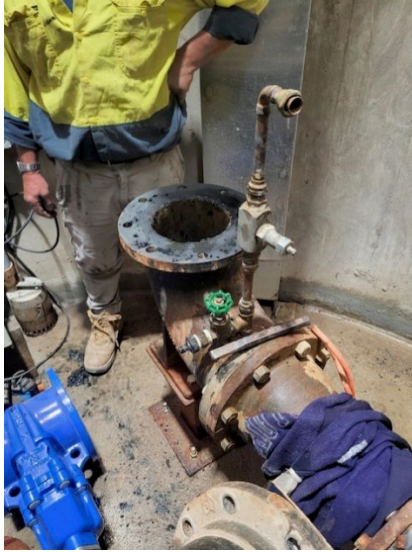
Change SV and non-return valves at No 2 Pump Murray St pumping station
